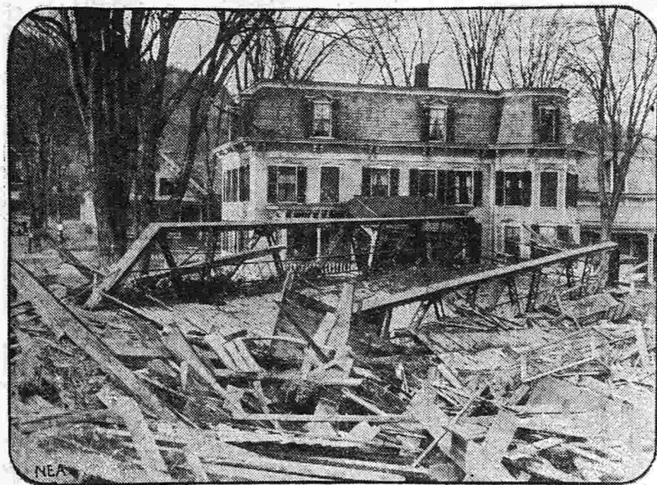
Occupants of this Montpelier, Vt., home found a badly smashed steel highway bridge on their porch when they awakened the morning of the flood. Ever see anything like it before?
